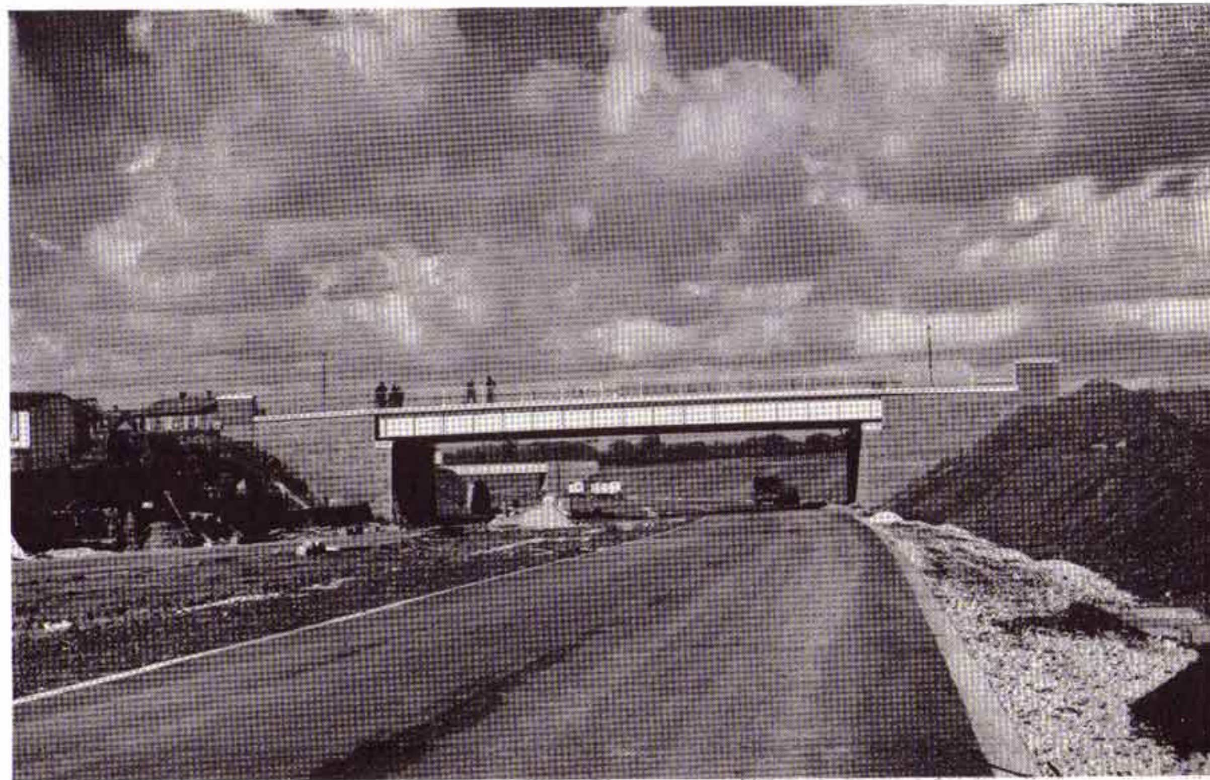
PLATE 7. LONGRIDGE ROAD BRIDGE.
