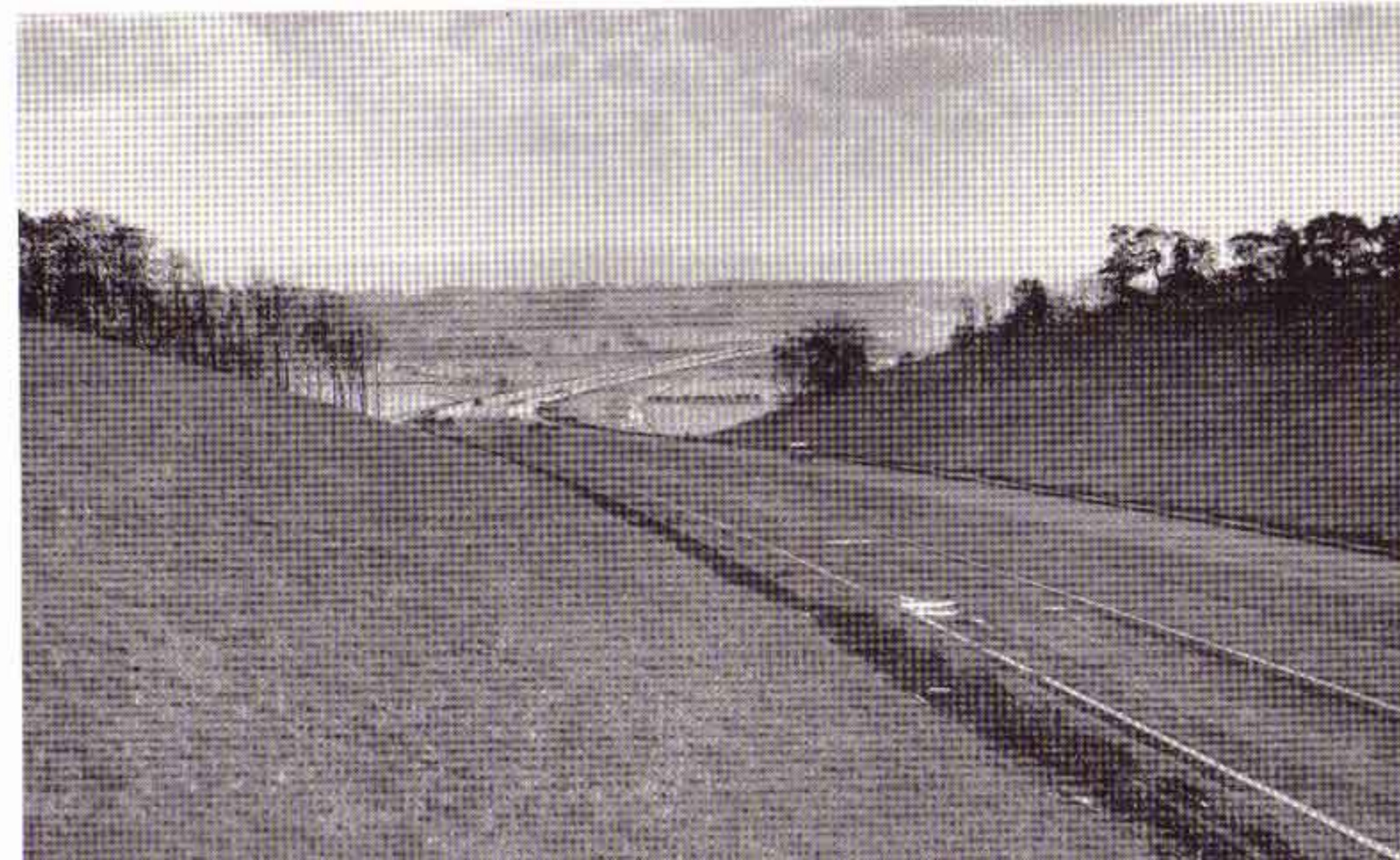
PLATE 6. NORTH ESCARPMENT TO RIBBLE VALLEY NEARING COMPLETION.
