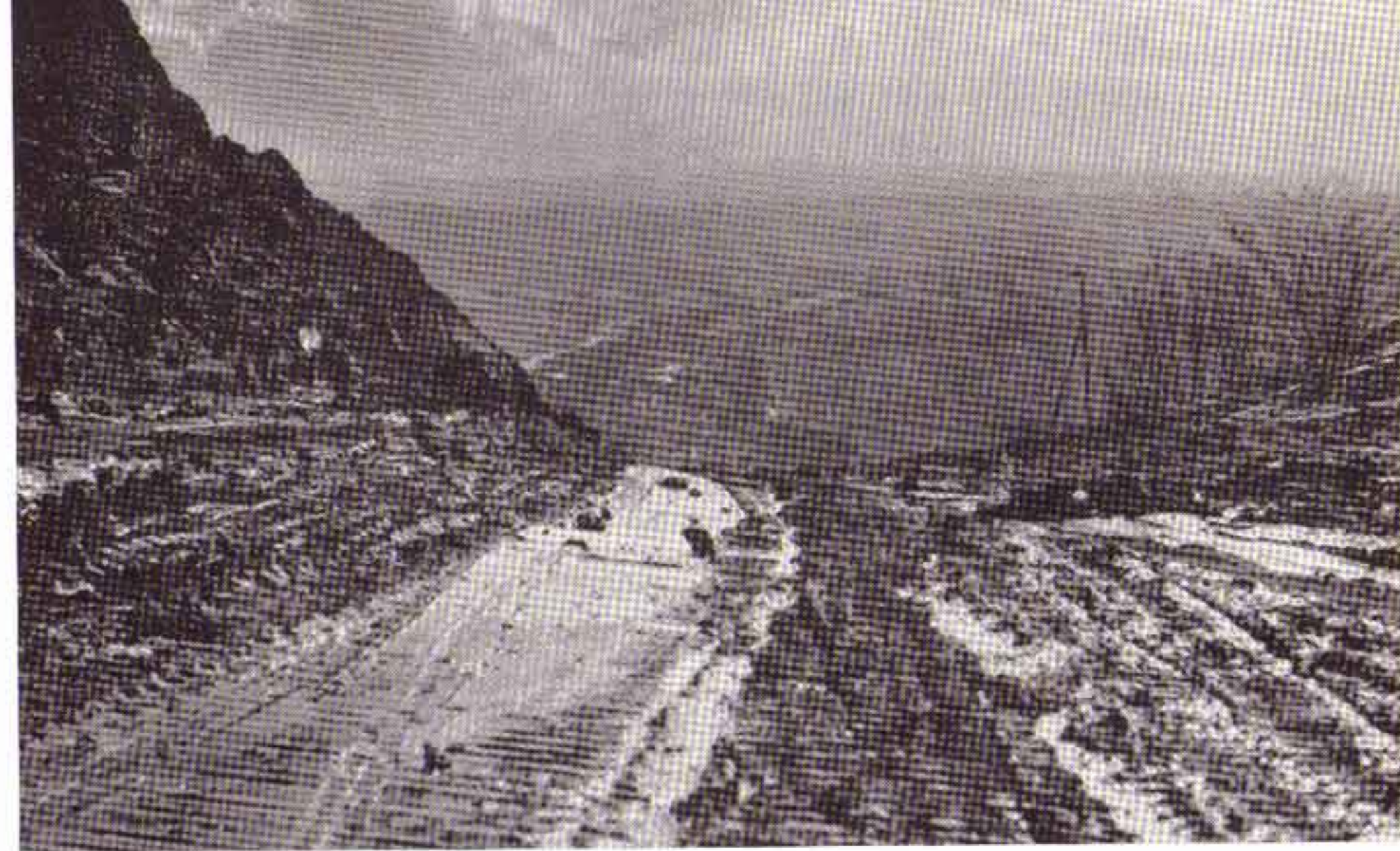
PLATE 5. NORTH ESCARPMENT TO RIBBLE VALLEY UNDER CONSTRUCTION.
