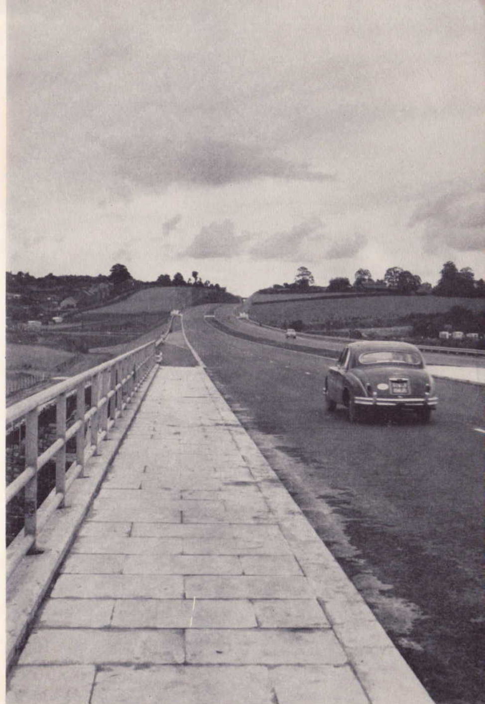
The undulating nature of the country is illustrated at this point where the Ross By-pass crosses the Wye and immediately enters a rock cutting 35 feet deep.
