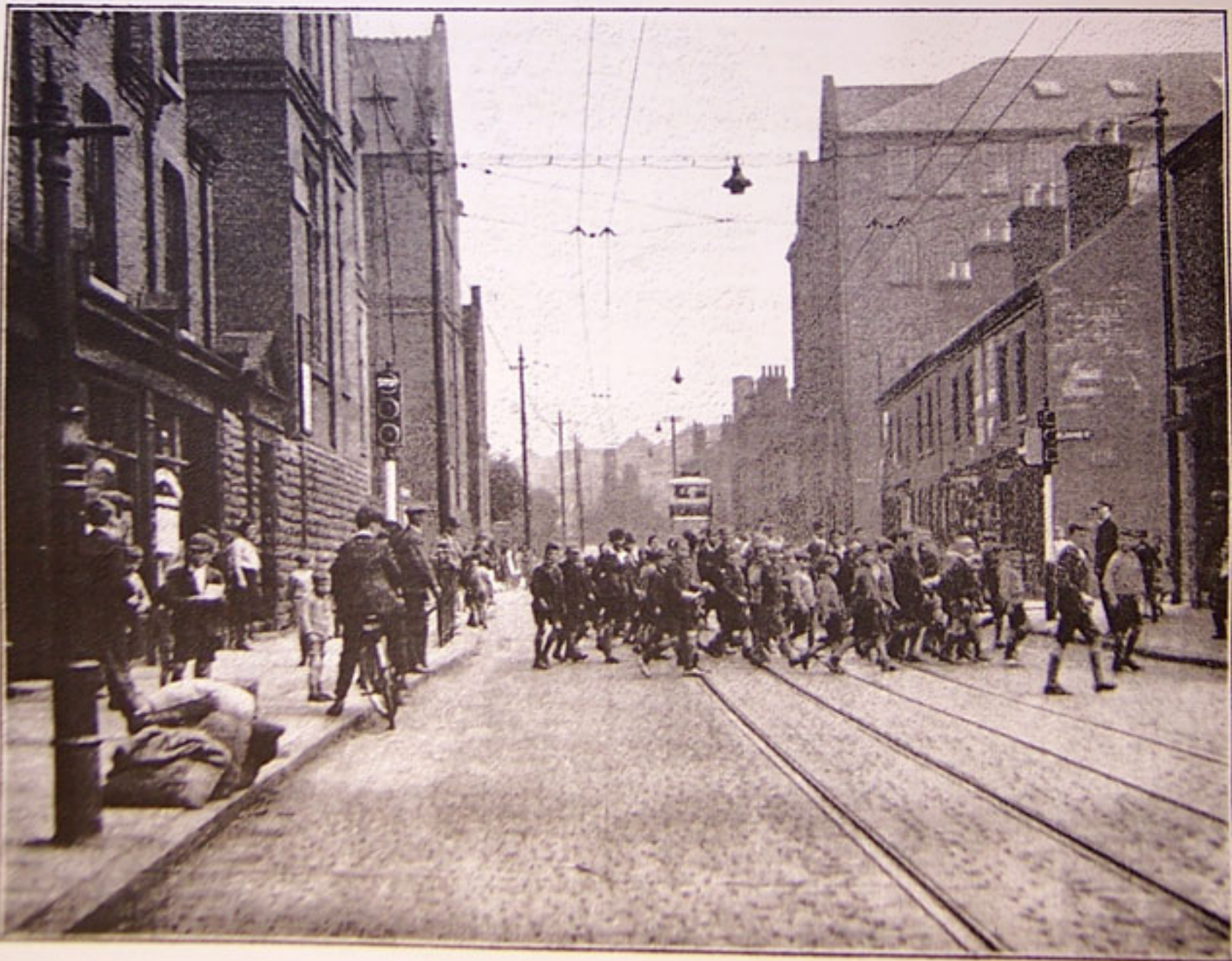
Crossing signal at school crossing.
